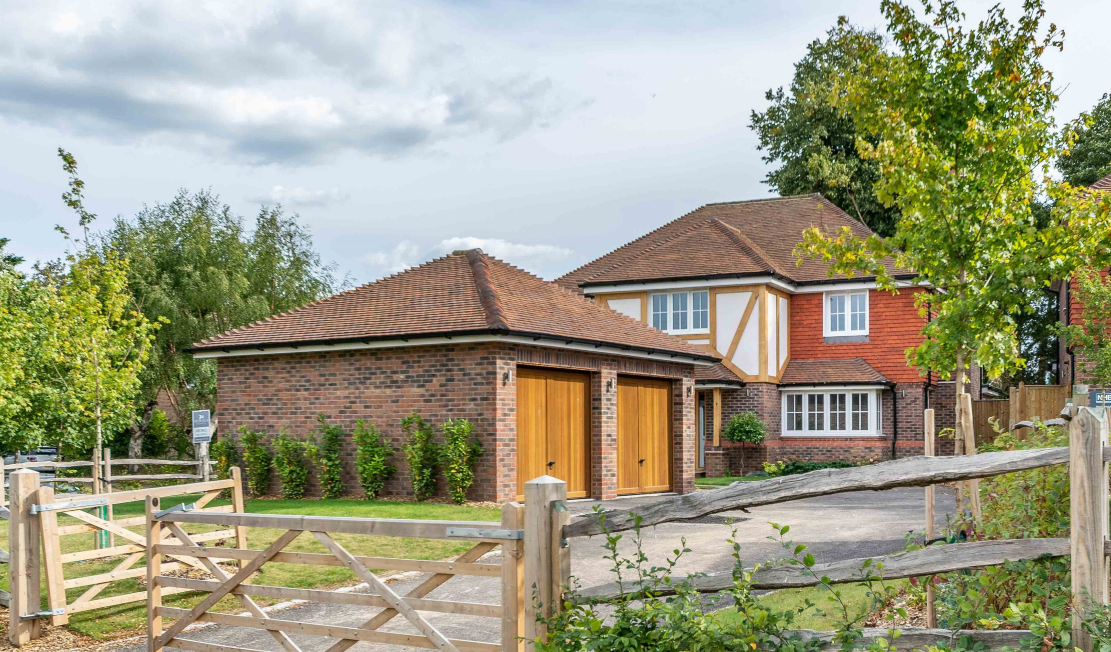
Oakhurst House West Drive, Angmering, West Sussex, BN16 4JE
